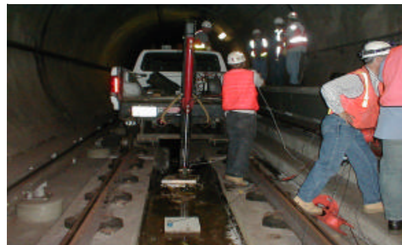
Figure 5 - Vibration test measurements in progress in MTA tunnel
