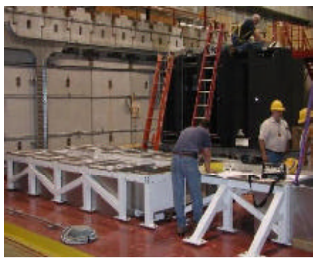
Fig. 4 - The Klystron Mounting Boxes on the Klystron/Modulator Support Stand.
