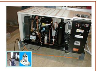
The chiller ( $\sim$ 700 lb) shown above vibrates by 2-3micron at 59Hz. If mounted rigidly, it transmits  $\sim$ 30nm to the floor near the support. Same chiller mounted on soft spring transmits considerably less vibration to the floor (<nm).
